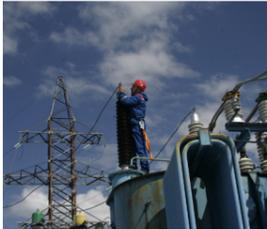
**2013** Substation 110kV Koksovaya. «EvrazEnergTrans» LLC Overhaul repair of electrical equipment at the Substation Koksovaya with replacement of linear high-voltage inputs to the Overhead transmission line Koksovaya 1,2 and T1
